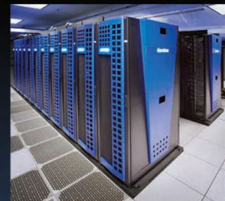
SDSC'S GORDON SUPERCOMPUTER. PHOTO: ALAN DECKER.
